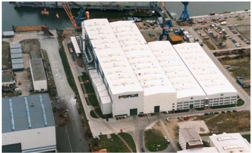
Picture: Caterpillar Motoren Rostock GmbH.
